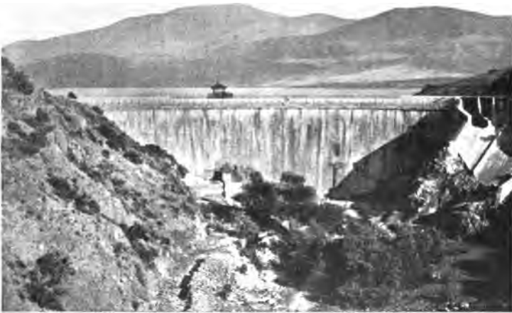
FIG. 116. — SWEETWATER RESERVOIR, NEAR SAN DIEGO, CALIFORNIA
